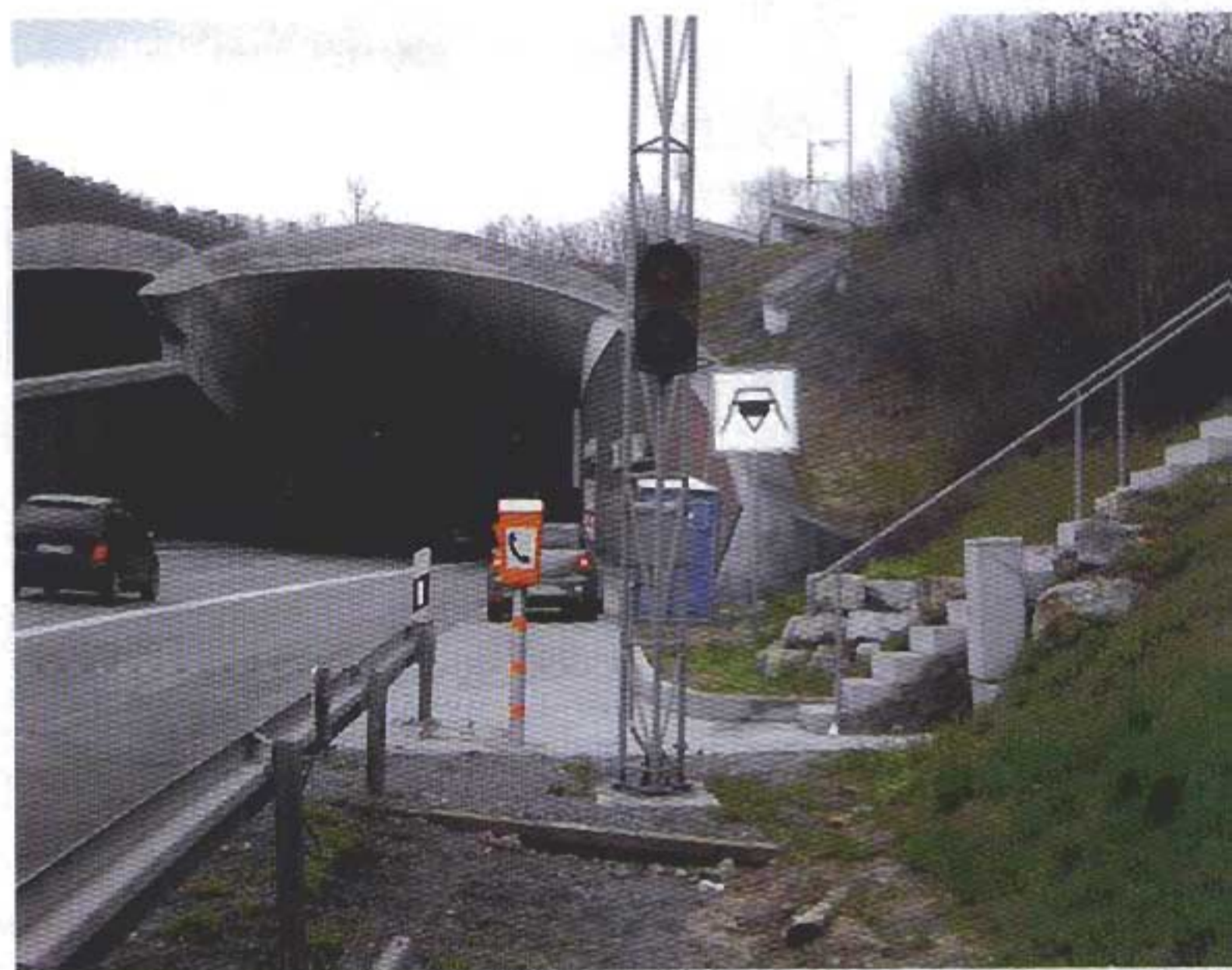
Entrance section of the newly renovated Kappelberg Tunnel, Germany.
